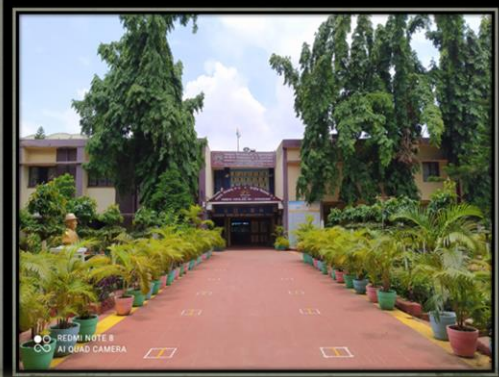
VIDYALAYA ENTRANCE GATE
